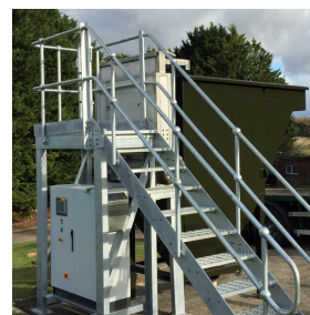
Fig. 4 Soneco® Sono-electrochemical water treatment for removal of Phosphorus from wastewater
