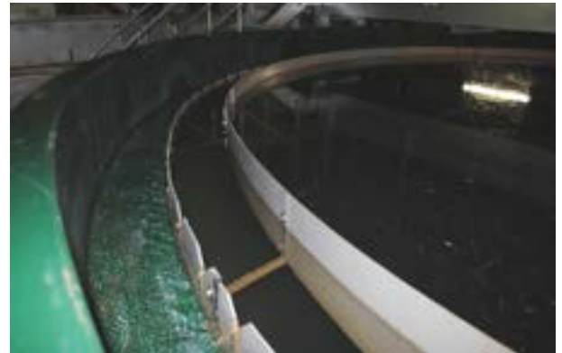
Final water holding tank. Water was tested prior to release to surface drinking water source
